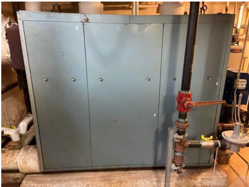
Smith Boiler Assembly – Cast Iron Sectional Boiler
