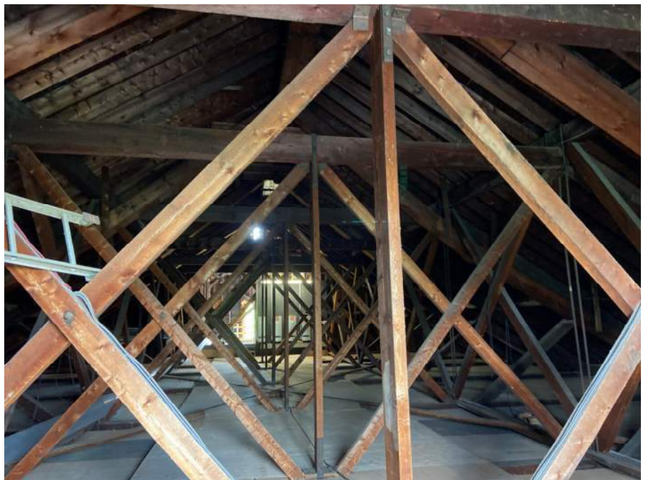
Sanctuary Attic Space
