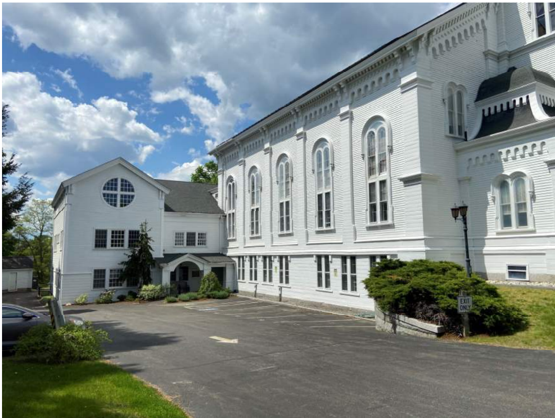
South Church – 2003 Parish Hall Addition and South Elevation of 1860 Sanctuary
