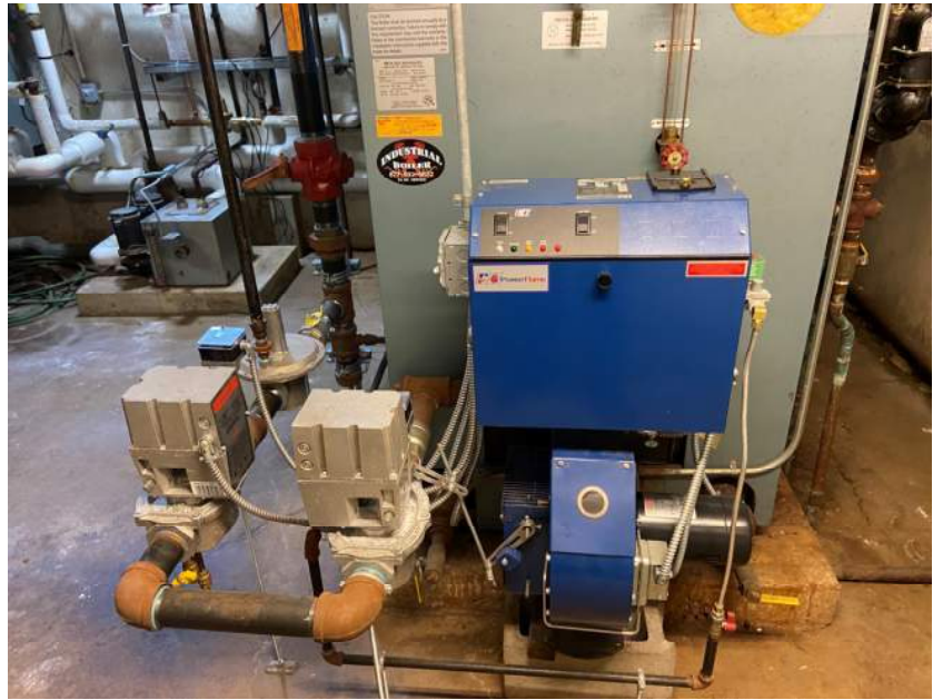
Power-Flame Gas Low-High-Low Boiler Burner
