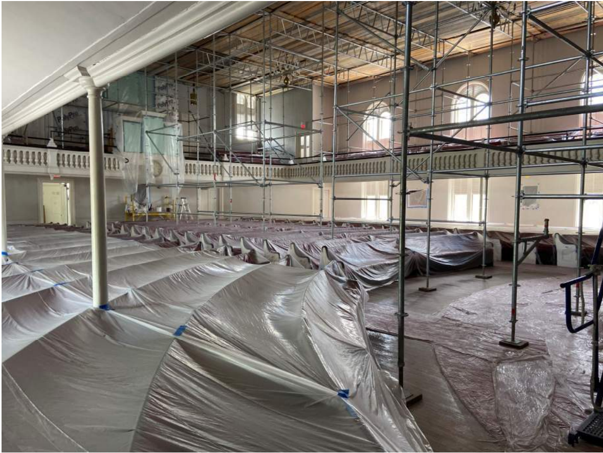
Sanctuary Space (Currently Undergoing Ceiling Plaster Repairs)
