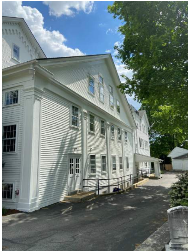
1956 & 2003 Addition West Elevation (Rear of Building)
