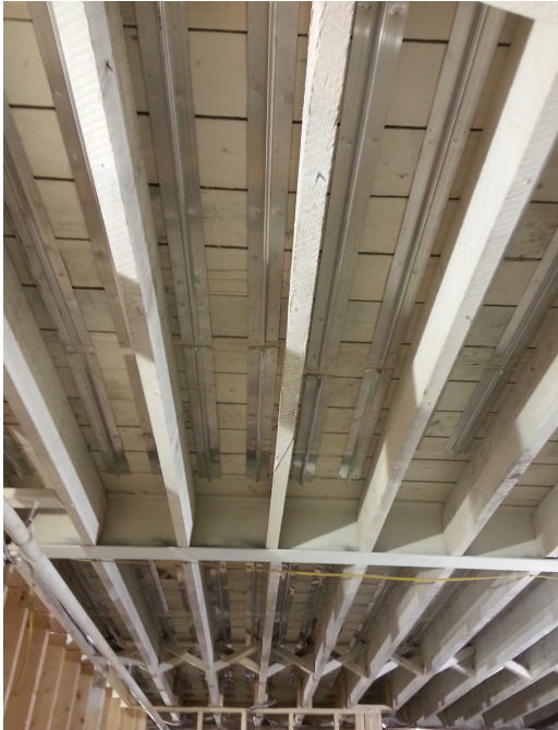
RADIANT "STAPLE-UP" SYSTEM
